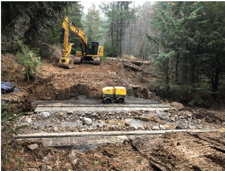
Photo 2. A simulated streambed was constructed between the two concrete footings. The slotted channel in the concrete footings on either side of the streambed that will hold the new culvert in place is clearly visible in this photo.
