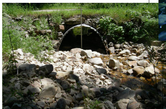
Undersized culvert at Langlois Creek Road Crossing, 2007.
