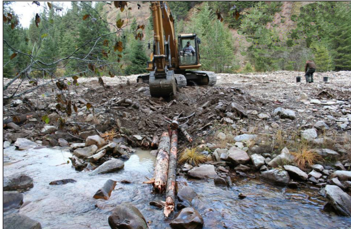
Installing logs and riparian plantings to enhance bank stability on the East Fork of Pine Creek, fall, 2008.
