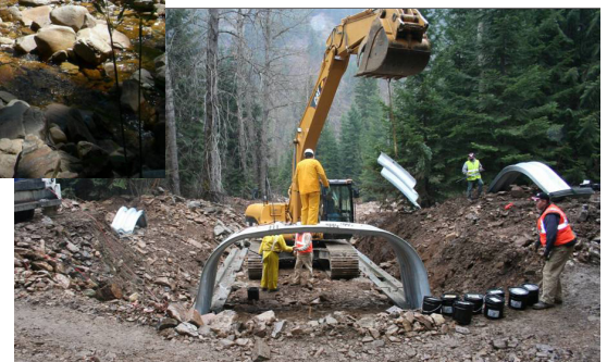
Installing replacement culvert at Langlois Creek, November 2007.
