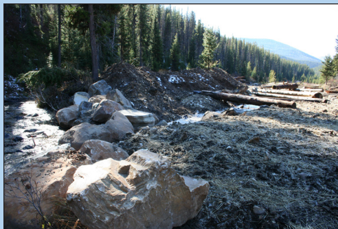
(10/29/08) Looking downstream - old channel on the left, new channel on the right, stockpiled soil in the middle for 2009 work. Temporary flow control intersection provides some flow to the new channel to help with revegetation, especially willow staking.
